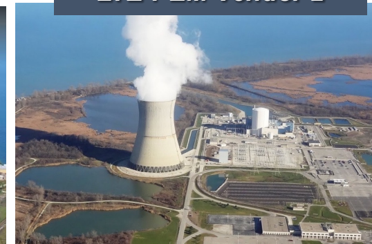
Davis-Besse Nuclear Power Plant LTE-PEM Vendor 2
