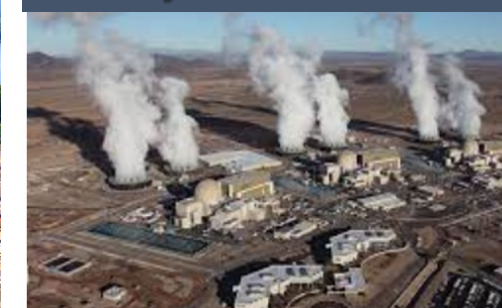
Palo Verde Gen Station Hydrogen Production for Combustion and Synthetic Fuels
